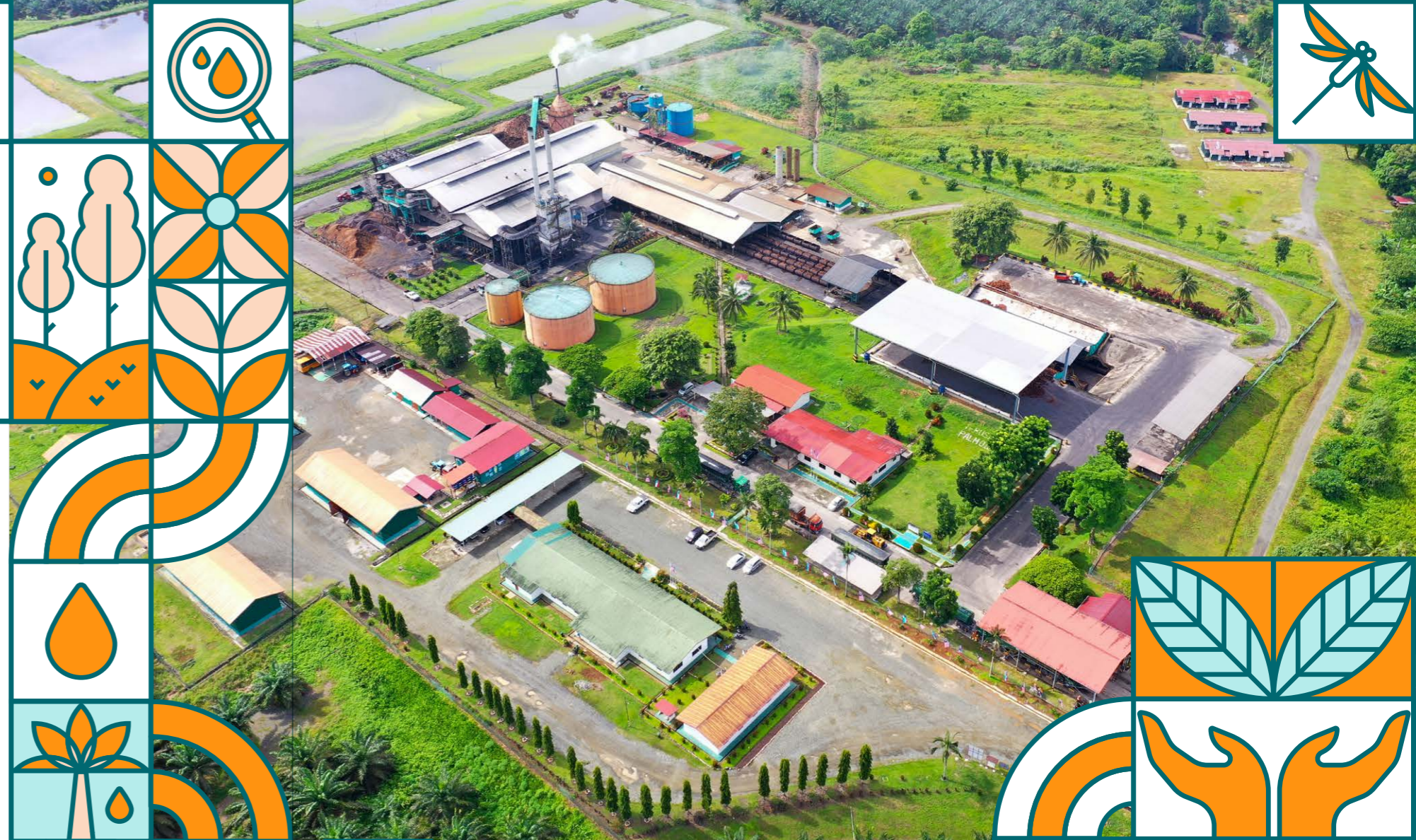
Wilmar palm oil mill in Sabah, Malaysia.
